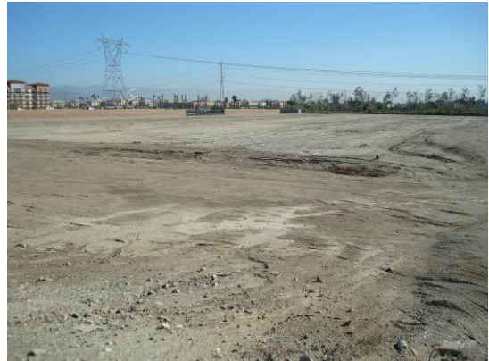
New ASR Wells Nos. 1 and 2 would be located at opposite ends of the proposed Foothill/Rochester reservoir site.
