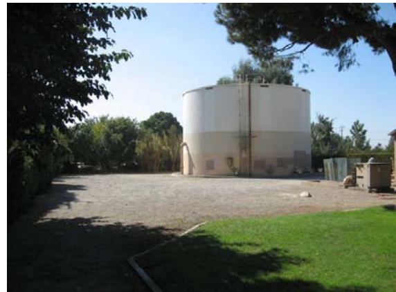
The Well No. 2 site has an existing steel reservoir, well, and electrical building.
