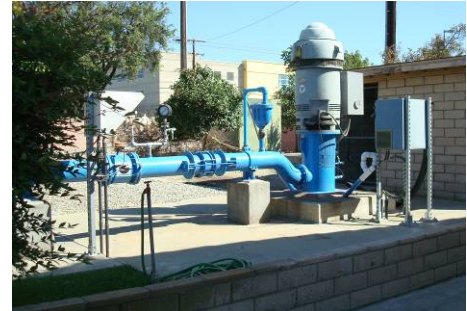
The New ASR Well design would be similar to the existing MVWD ASR Well No. 4, as shown.
