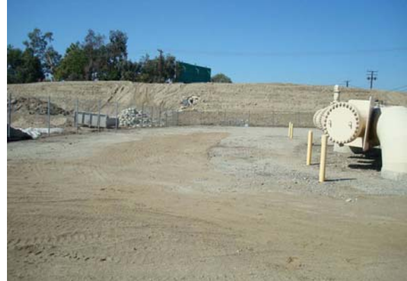
The New ASR Well would be located on the south west corner of the property.
