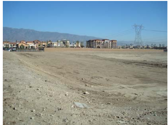
Future Site of Ontario's Two 8 MG Reservoirs
