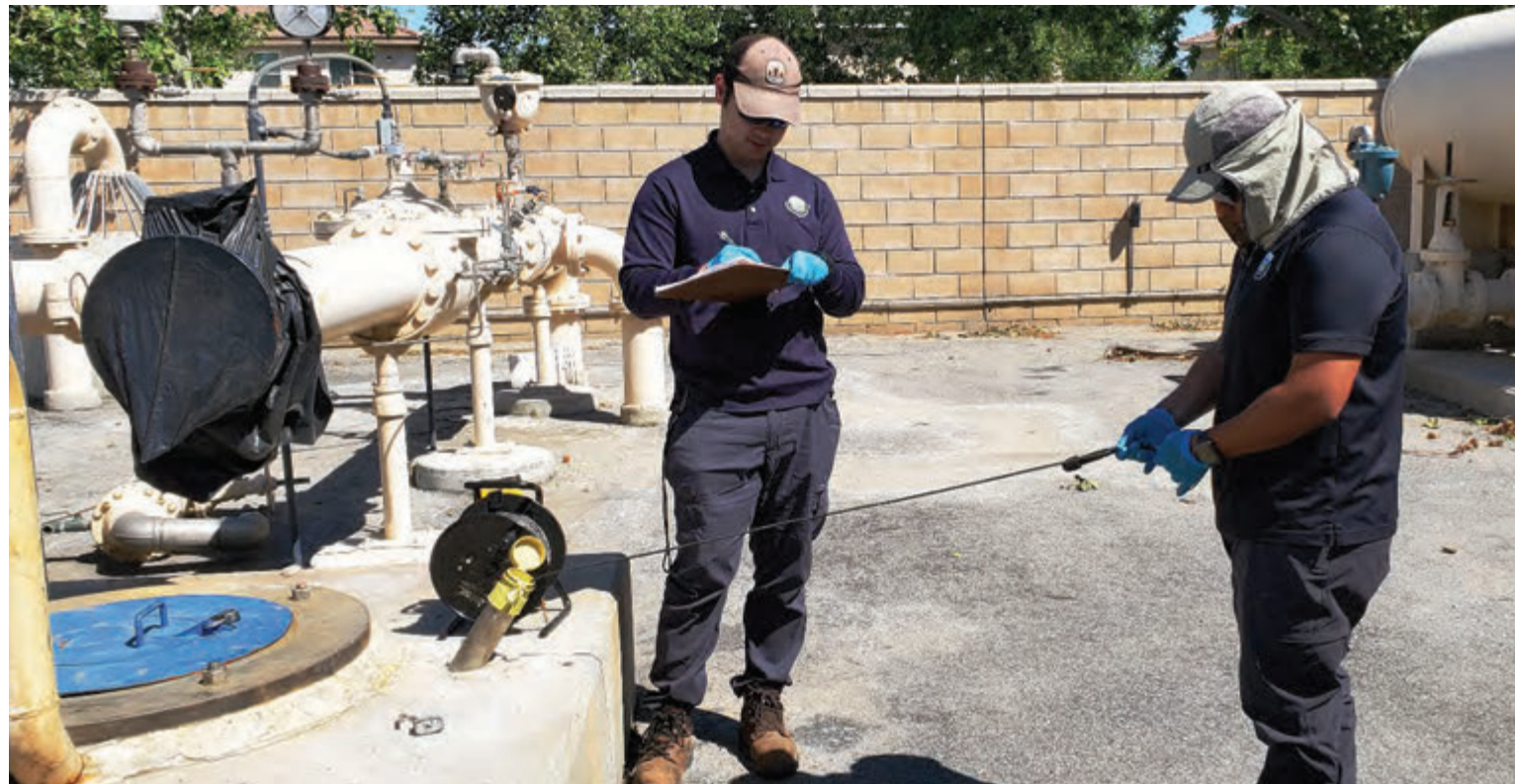
Downloading transducer data to track water levels in the Basin
