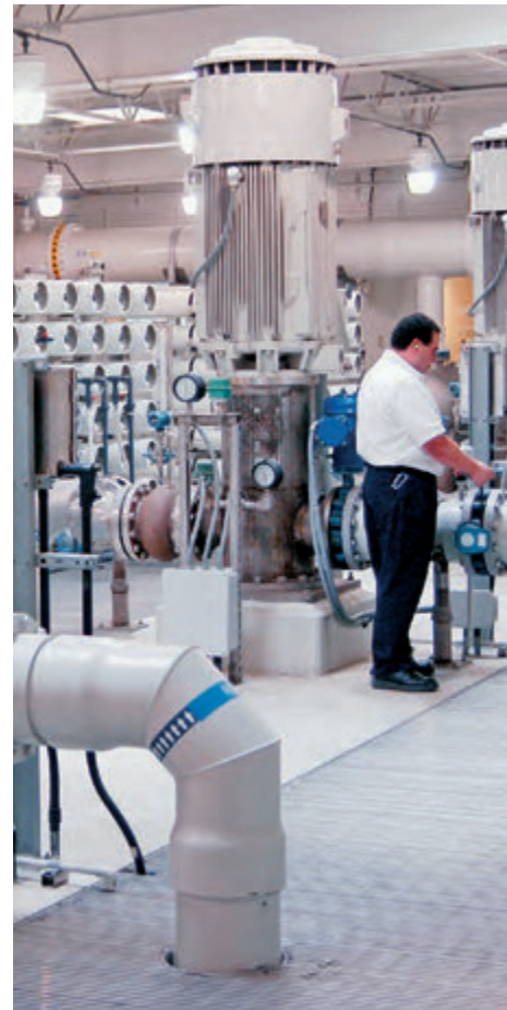
The treatment processes at the Chino I and Chino II Desalters include reverse osmosis and ion exchange for removal of nitrate and total dissolved solids.
