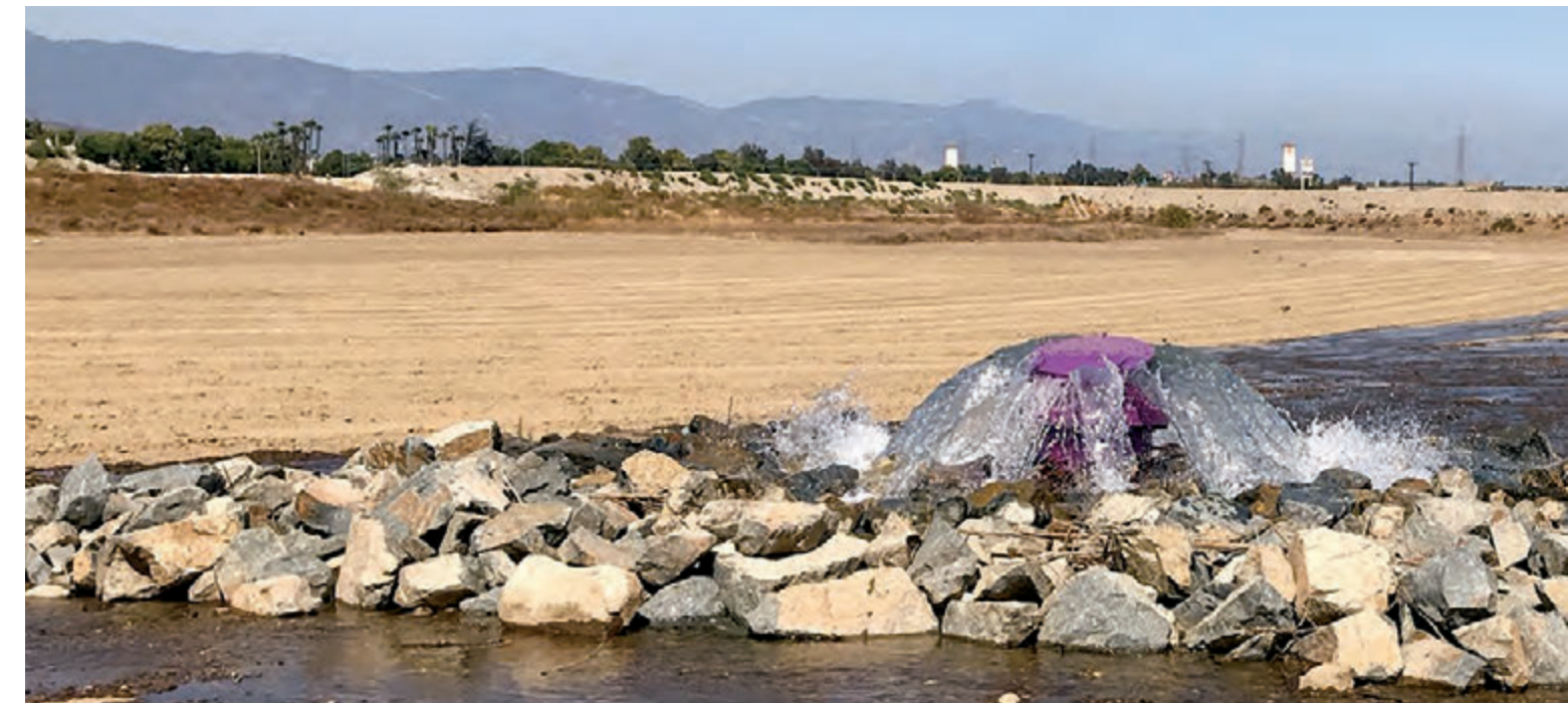
Recycled Water is now being recharged into the San Sevaine Basin as a result of the RMPU capital improvements.
