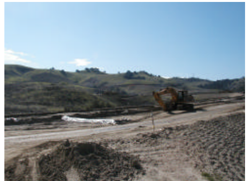
Construction of Oak Crest Golf Course in Chino Hills
