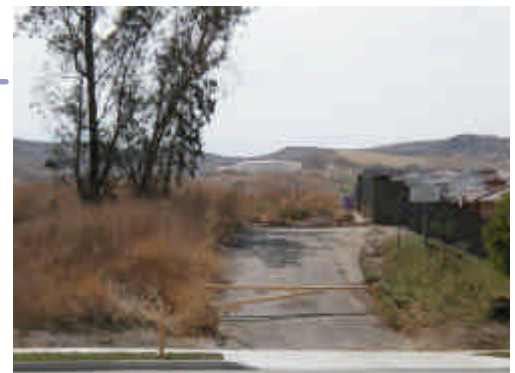
3 MG Recycled Water Reservoir in Chino Hills
