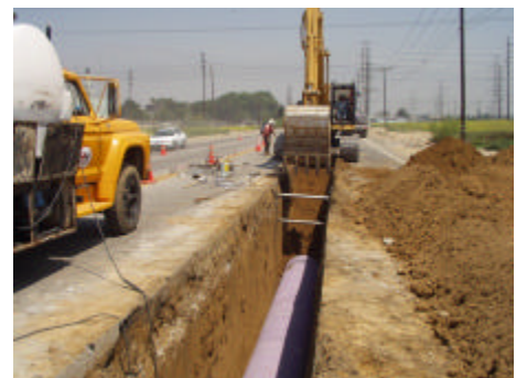
Phase I Etiwanda Recycled Water Pipeline
