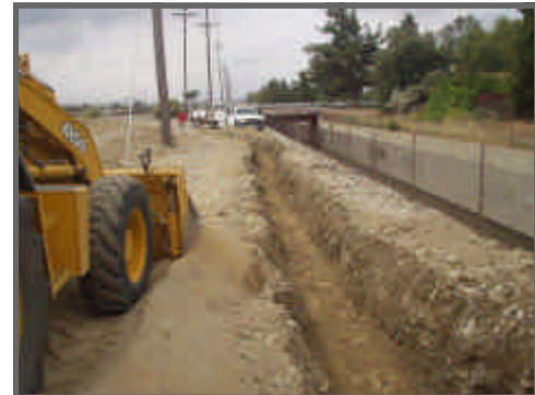
Montclair Basin Trenching for SCADA
