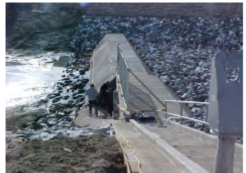
Banana Basin-Sluice Gate Structure
