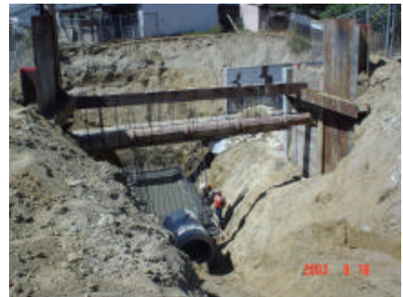
Brooks Basin San Antonio Channel Water Diversion Pipeline
