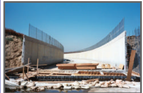
Turner 2,3,& 4- Deer Creek Drop Inlet Structure
