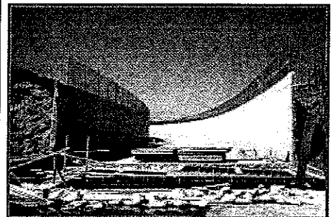
Turner 2,3,& 4- Deer Creek Drop Inlet Structure
