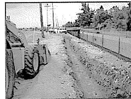
Montclair Basin Trenching for SCADA
