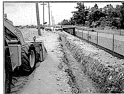
Montclair Basin Trenching for SCADA
