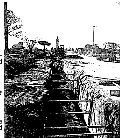
Edison Avenue Pipeline
