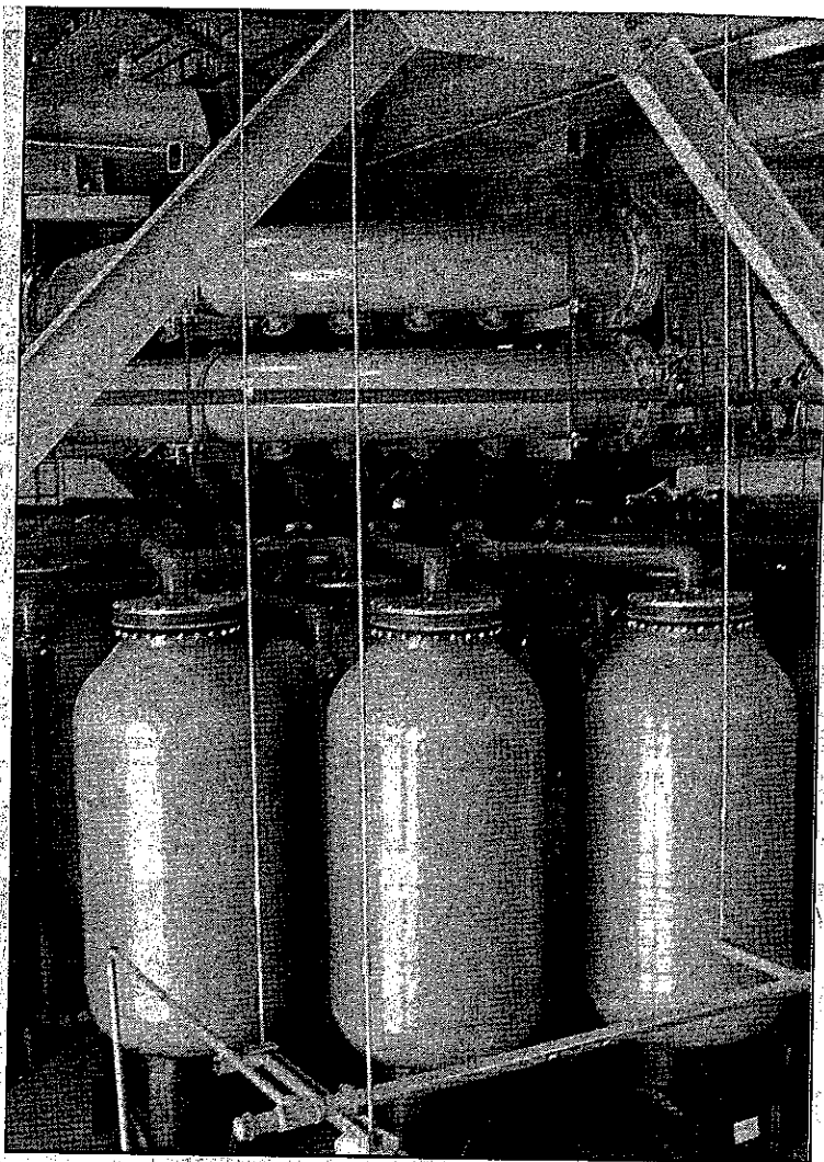
Champion photo by Richard Block Inside Chino's new water treatment plant, these vessels filter nitrates and perchlorate from well water.
