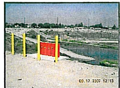
Lysimeters at 8th Street Basin
