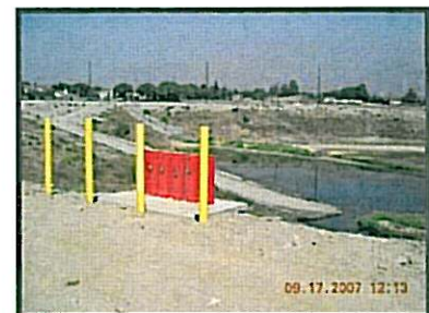
Lysimeters at 8th Street Basin
