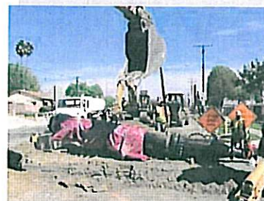
San Antonio Channel Pipeline Construction
