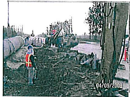
1630 Segment A Pipeline Construction
