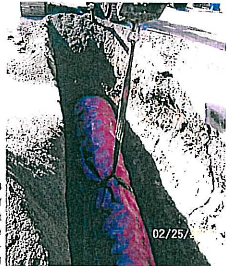
San Antonio Channel Segment B Pipeline
