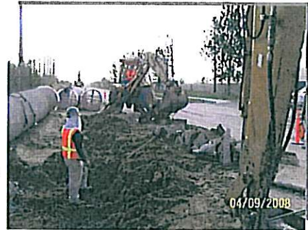
1630 Segment A Pipeline Construction
