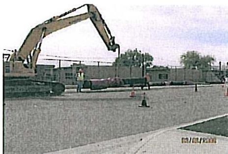
San Antonio Channel Segment B Pipeline
