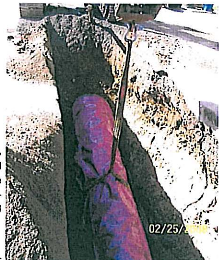
San Antonio Channel Segment B Pipeline
