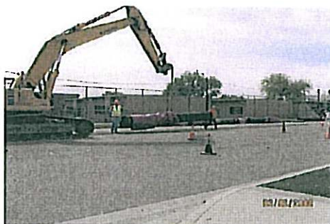
San Antonio Channel Segment B Pipeline
