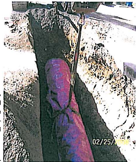
San Antonio Channel Segment B Pipeline
