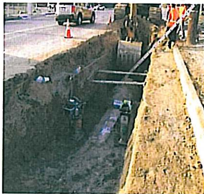
San Antonio Channel Segment B Pipeline
