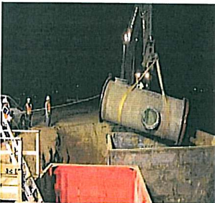
San Antonio Channel Segment B Pipeline
