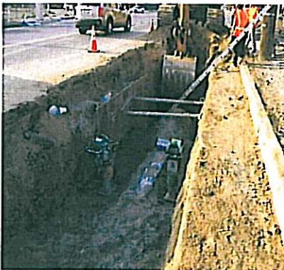
San Antonio Channel Segment B Pipeline
