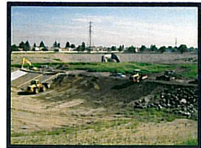
Construction of Berm No. 1 at Declez
