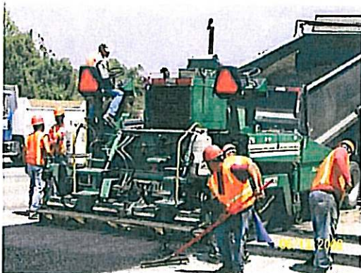
North Etiwanda Recycled Water Pipeline Segment B
