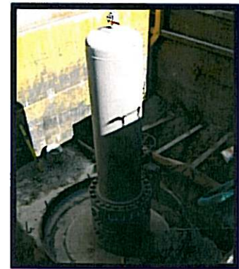
Valve installed at CB-14
