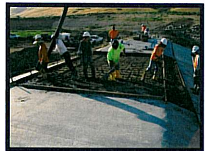
Construction Concrete Spillway at Declez
