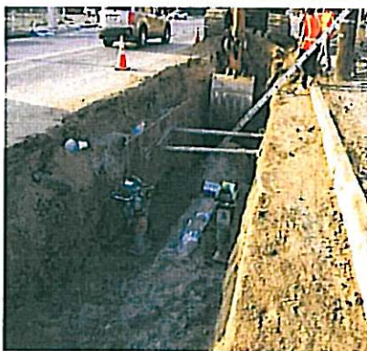
San Antonio Channel Segment B Pipeline
