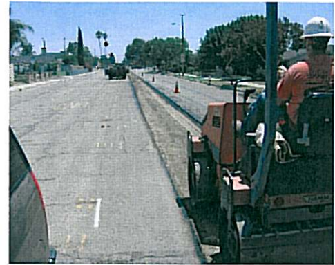
WRO4446 San Antonio Channel Pipeline, Segment B
