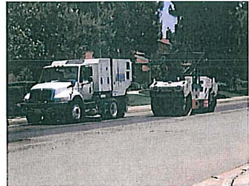
San Antonio Channel Pipeline, Segment B
