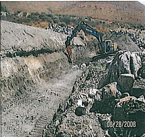
Chino Basin Facilities Improvements Phase II
