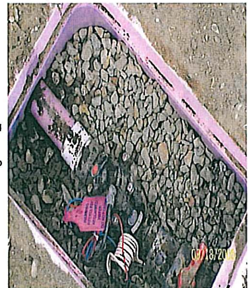
Ontario and MVWD Public Schools Retrofit
