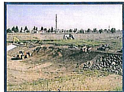
Construction of Berm No. 1 at Declez
