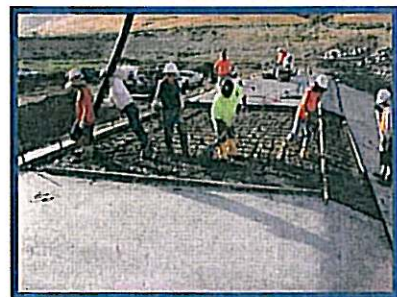
Construction Concrete Spillway at Declez
