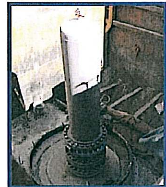
Valve installed at CB-14
