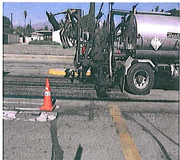
San Antonio Segment B: Paving Improvements on Orchard St in Montclair.
