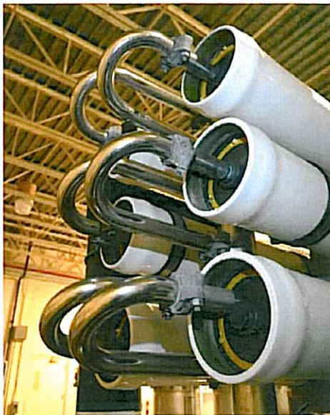
Reverse osmosis equipment used in desalting facilities.
