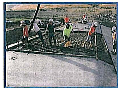
Construction Concrete Spillway at Declez
