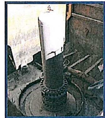
Valve installed at CB-14
