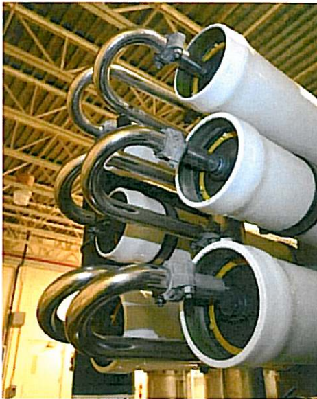
Reverse osmosis equipment used in desalting facilities.
