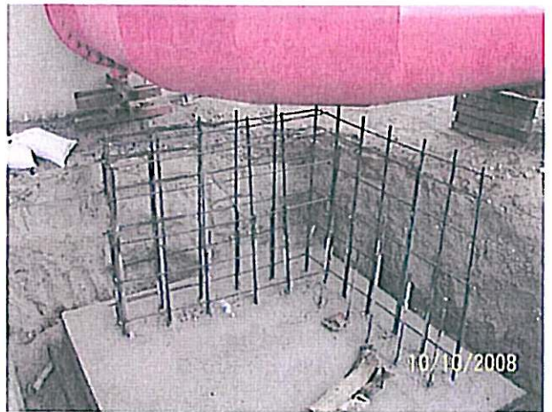
1158 Zone Reservoir upgraded pipe support Foundation
