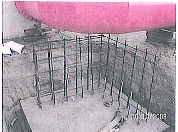
1158 Zone Reservoir upgraded pipe support Foundation
