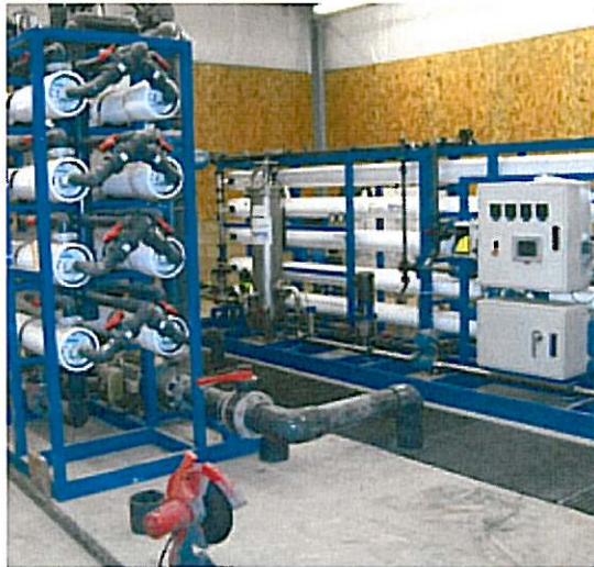
Photo: Tom Stewart Highly purified RO is one step in the process to turn wastewater into a purified product.
