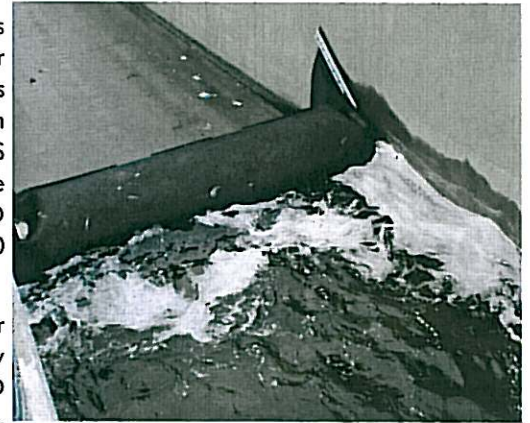
Rubber Dam in action
