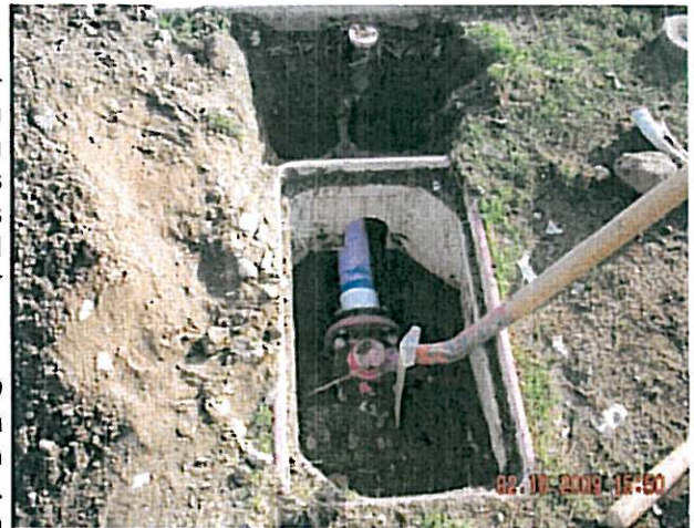
Vineyard Elementary School, City of Ontario
