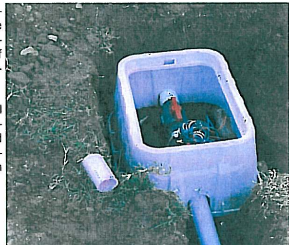
Corona Elementary School, City of Ontario
