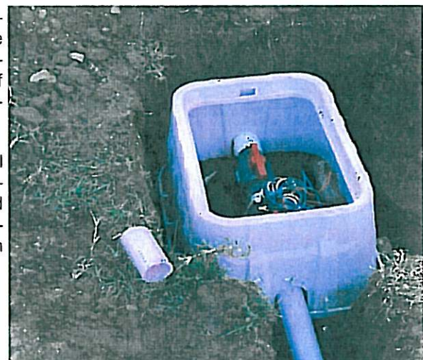
Corona Elementary School, City of Ontario
