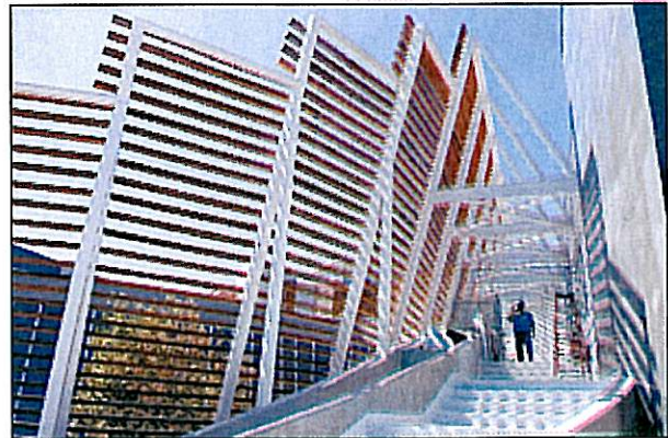
A trellis made of wood planks recycled from Filippi Winery wine barrels shades the staircase at the Frontier Project building in Rancho Cucamonga. The building is designed to be energy-efficient and environmentally friendly. (Jennifer Cappuccio-Maher/Staff Photographer)
