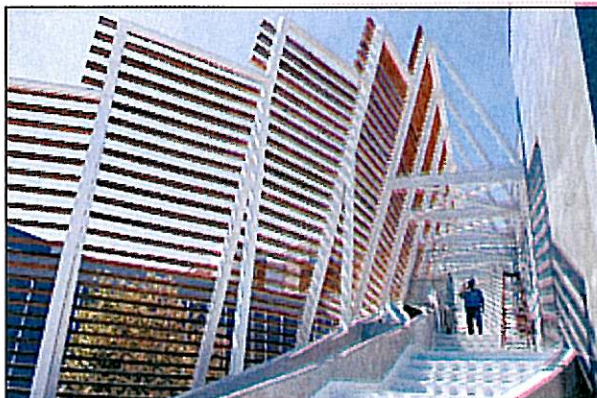
A trellis made of wood planks recycled from Filippi Winery wine barrels shades the staircase at the Frontier Project building in Rancho Cucamonga. The building is designed to be energy-efficient and environmentally friendly. (Jennifer Cappuccio-Maher/Staff Photographer)
