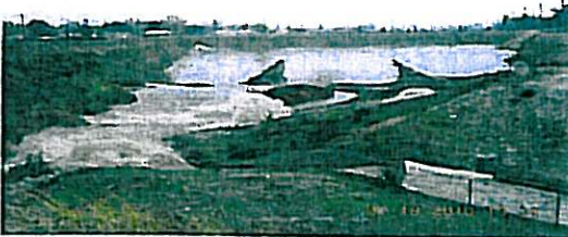
Storm Water-Montclair Basin
