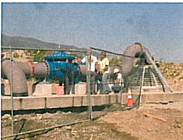
Installation of CB-14 Turnout
