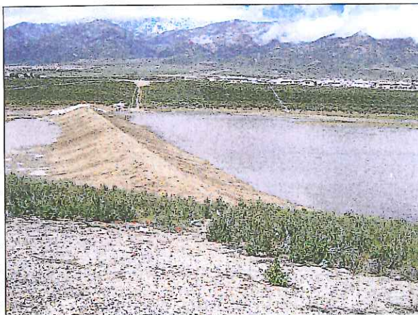
New San Sevaine Basin No. 5 Conservation Berm
