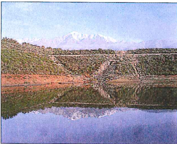
Lower Day Basin after a storm
