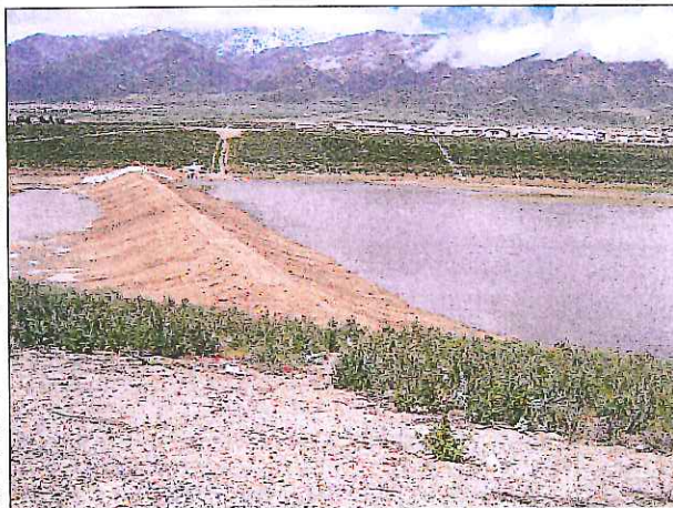
New San Sevaime Basin No. 5 Conservation Berm
