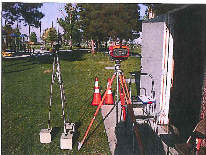
MZ-1 Monument Construction & Surveying
