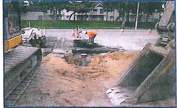
1299 E RW Pipeline – Air Vac Installation
