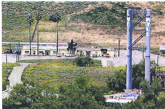
2003 / The Press-Enterprise Interim measures to clean up the former Wyle Labs site include wells that can extract contaminants, with the actual cleanup to begin next year. Six more wells are expected to be under construction by the end of the year.
