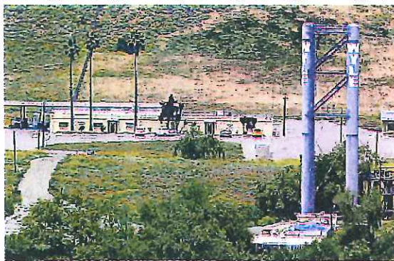
2009 / The Press-Enterprise Interim measures to clean up the former Wyle Labs site include wells that can extract contaminants, with the actual cleanup to begin next year. Six more wells are expected to be under construction by the end of the year.
