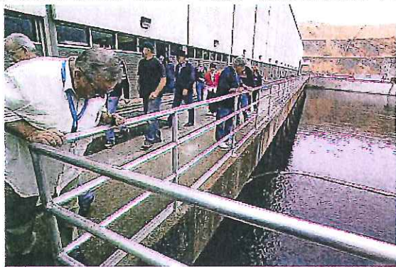
Los Angeles County Board of Supervisors field inspector Dickie Simmons checks out the Banks Pumping Plant at the start of the California Aqueduct during an inspection trip of The State Water Project.
