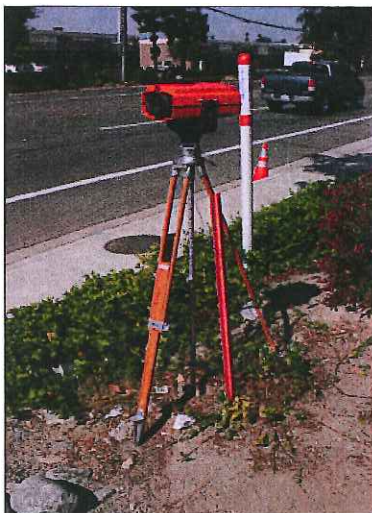
MZ-1 Monument Construction & Surveying
