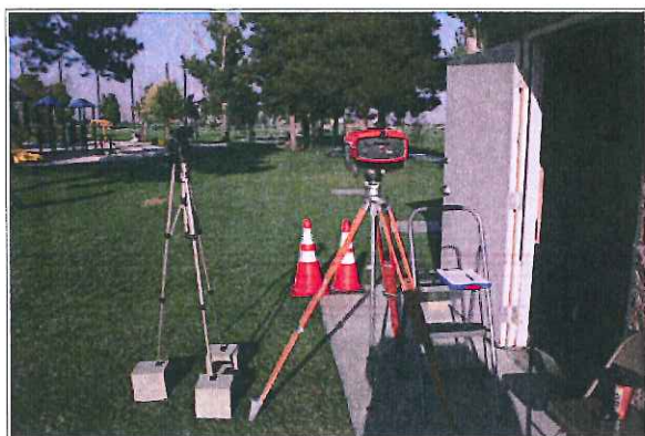
MZ-1 Monument Construction & Surveying
